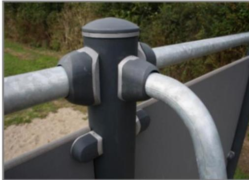
The connectors are made of die-cast aluminium, specially alloyed for the outdoor environments and heavy usage. The screws attaching the connectors are stainless steel and protected by zinc washers.
