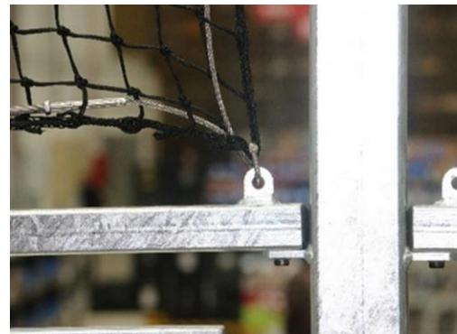
The net is made of a Ø4mm black polypropylene, better known as Nylon, with a mesh size of 45 x 45mm and reaches till 5m high. The nets will keep all balls in the MUGA and retains the transparency.
